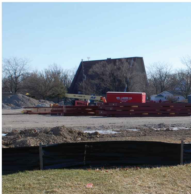
Progress on construction can be followed by visiting the webcam at www.defianceathletics.com/facilities/fhconstruction .
